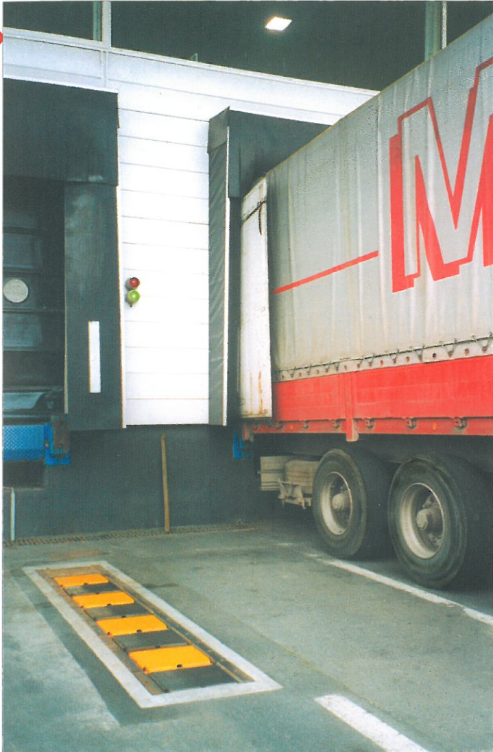
Truck restraint in neutral position. The traffic light signal shows green.
