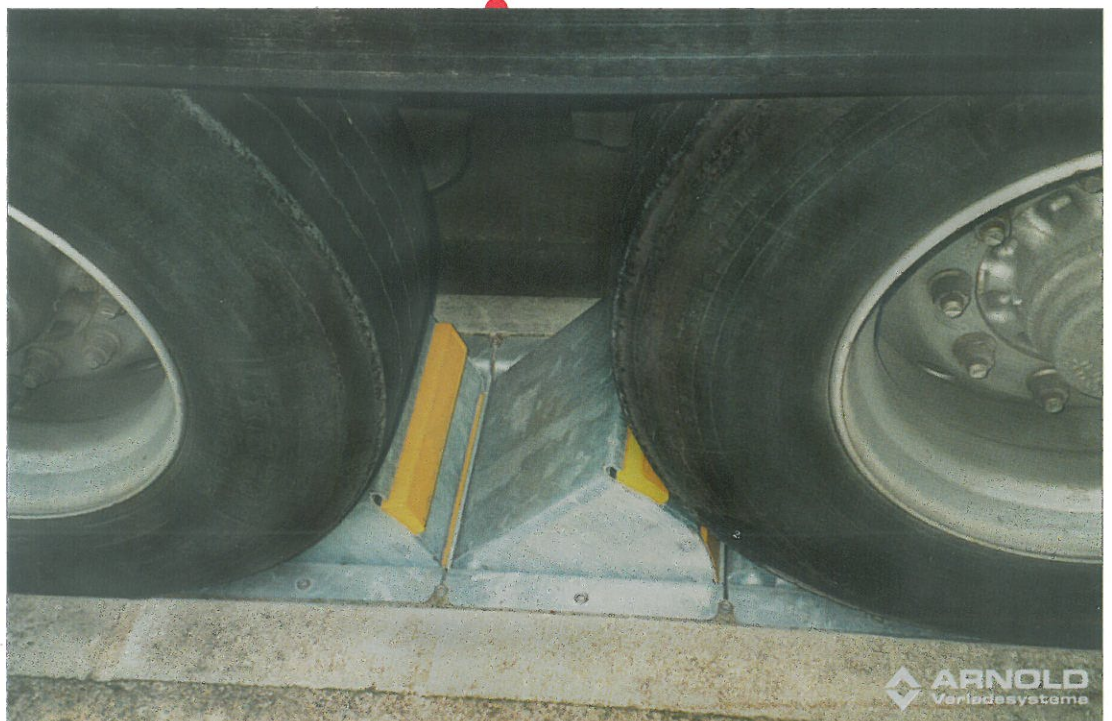
Truck restraint in neutral position. The traffic light signal shows green.
